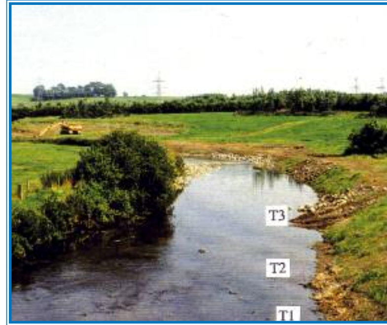
After rehabilitation works
